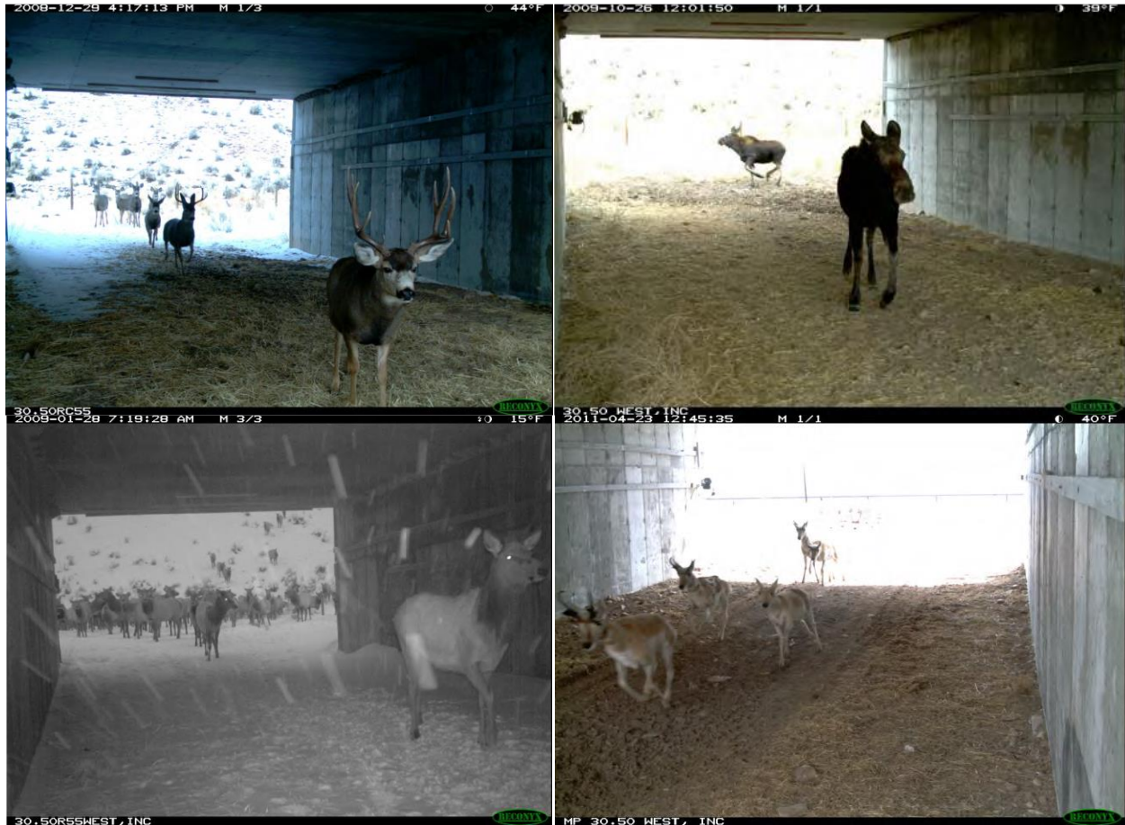
Figure 27. Movement of Mule Deer, Moose, Elk and Pronghorn Through a Wildlife Underpass in Nugget Canyon on U.S. Highway 30 west of Kemmerer, WY (Western EcoSystems 2011)
