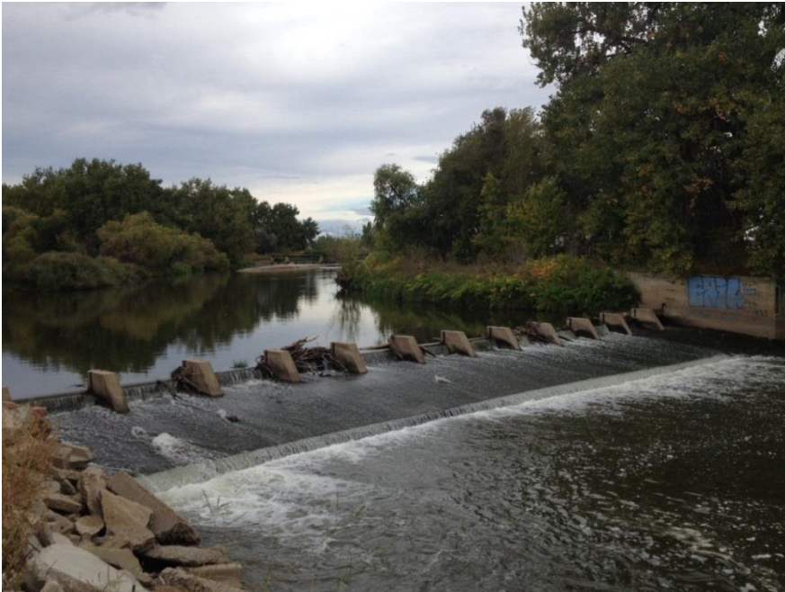
Figure 34. Existing B.H. Eaton Ditch Diversion Structure with Whitney Diversion in Background
