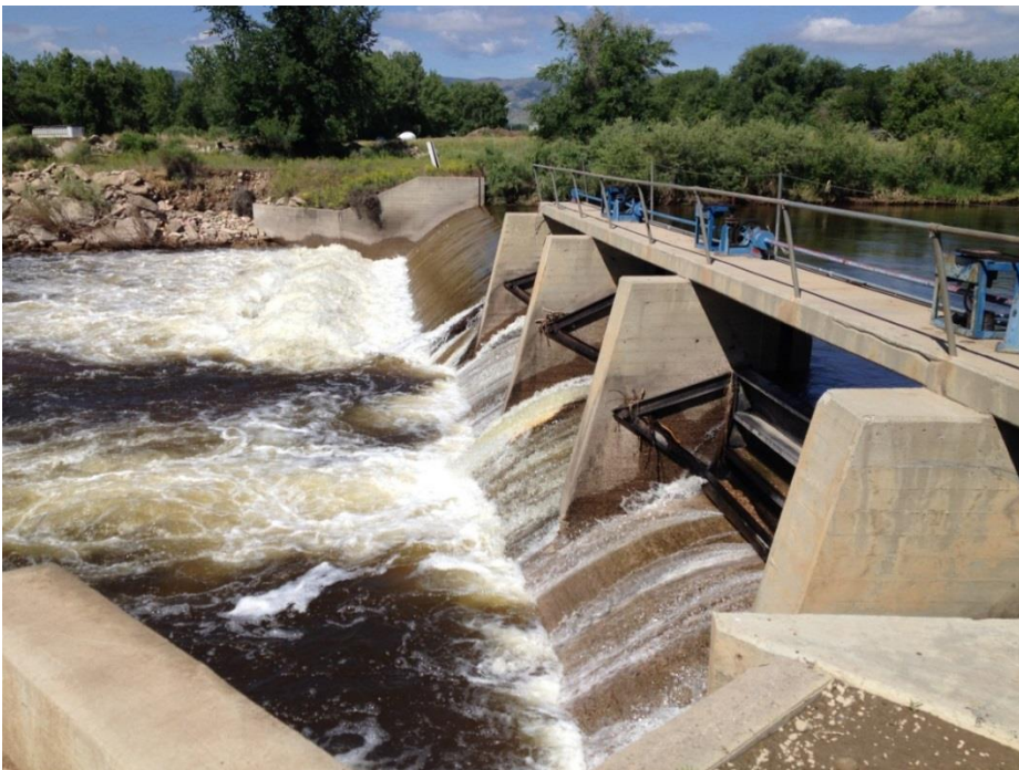
Figure 32. Existing Larimer-Weld Diversion Structure
