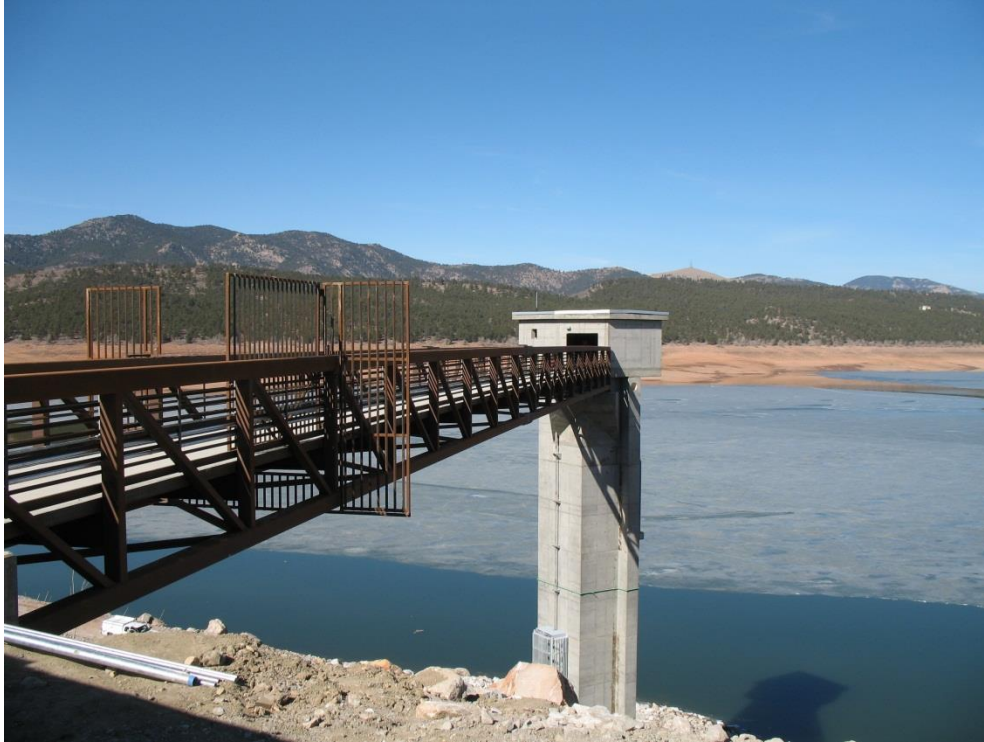
Figure 8. Multi-Level Outlet Tower at Carter Lake
