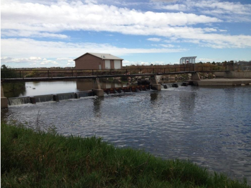
Figure 33. Existing Whitney Ditch Diversion Structure
